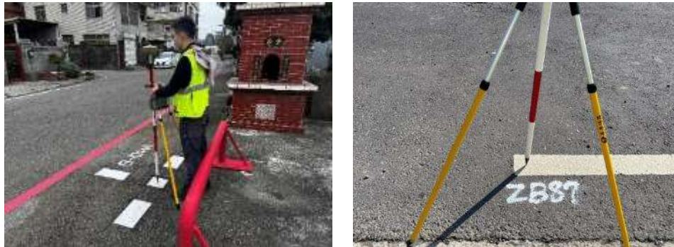
Figure 5. Newly established control points surveying
